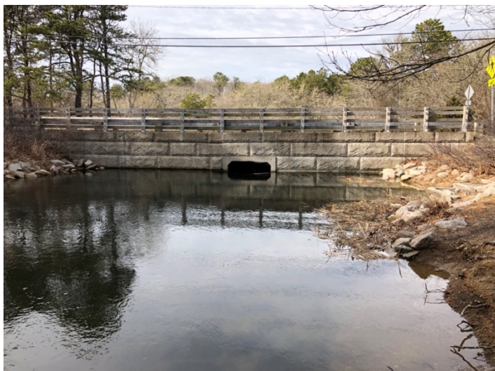
The current bridge and culvert at Crab Creek/North Dennis Road
